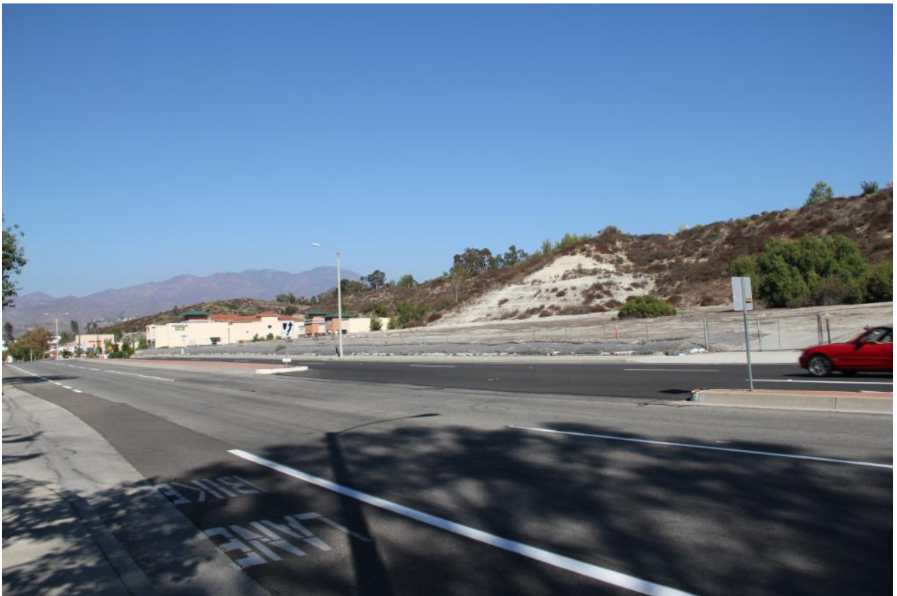
Possible site on LF Drive
